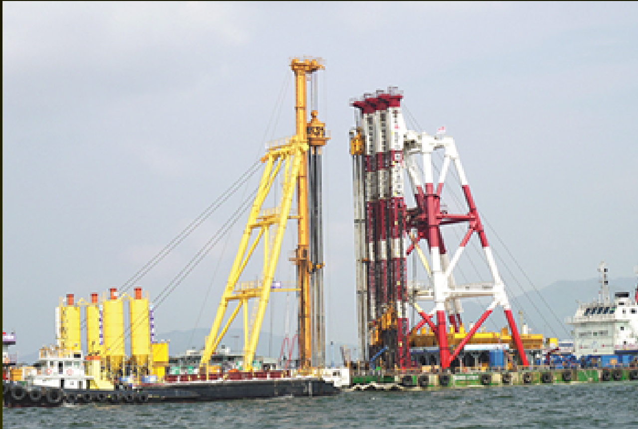
Barges for Deep Cement Mixing used in 3RS
