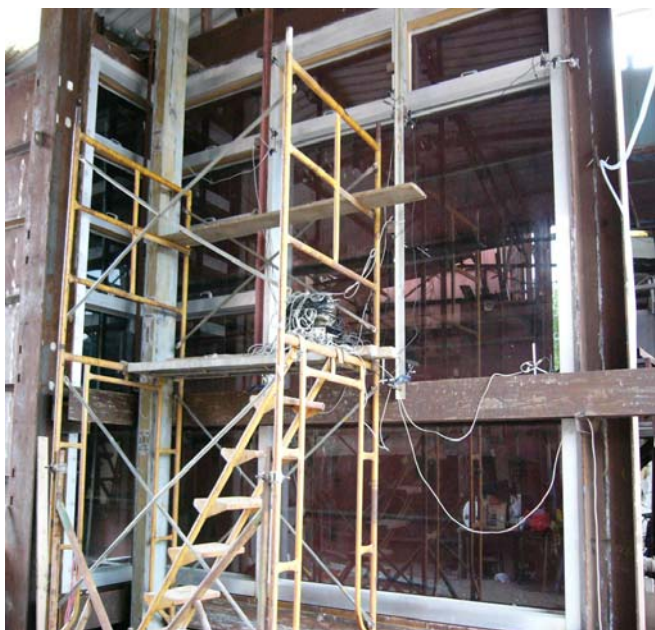
A curtain wall mock-up is ready for tests
