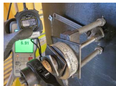
Pull-out test for anchor bolt
