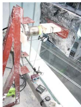
Load test on glass balustrades
