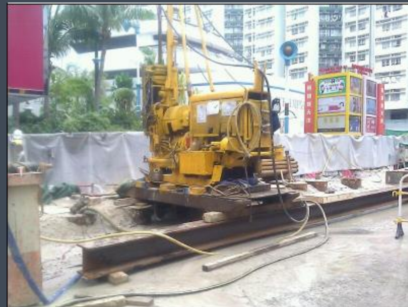
Drilling location in between the pipe piles
