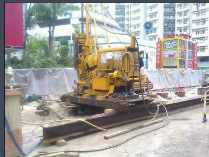
Drilling location in between the pipe piles
