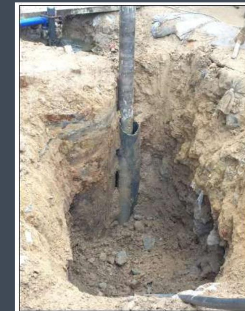
Damaged 220V buried live electric cable
