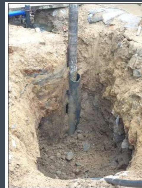
Damaged 220V buried live electric cable
